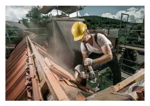
The vision of the cordless construction site has become reality: The new 36 Volt cordless angle grinder from Metabo is extremely powerful and, thanks to the completely encapsulated brushless motor with overload protection, also particularly robust and durable even in dusty environments and during the most demanding applications. Photo: Metabo
