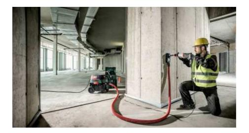
The KHE 2860 Quick combination hammer in use on a major construction site: Professionals drill holes in concrete up to 28 mm diameter in concrete with the new tools. All new rotary hammers can be combined with an extensive range of accessories: here with core bit for diameters up to 68 millimetres and with dust extraction. Photo: Metabo
